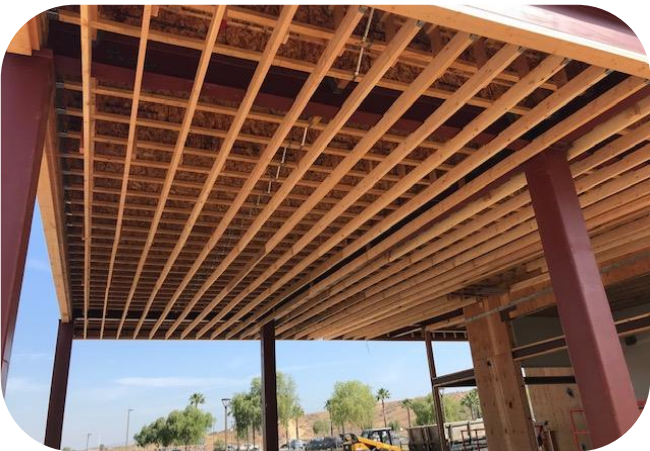
Patio Joist Installation
