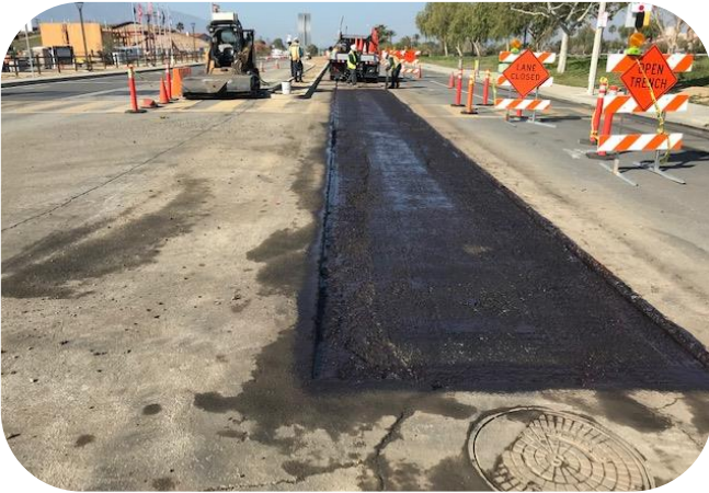
3rd Street Asphalt Prep
