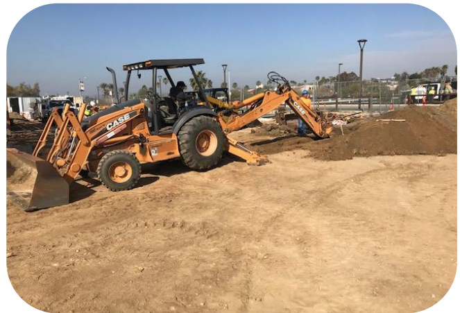
On site domestic water line trenching
