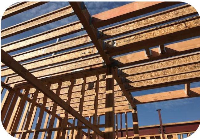
Roof joists/framing
