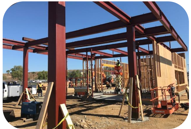
Structural steel and wall framing ongoing.
