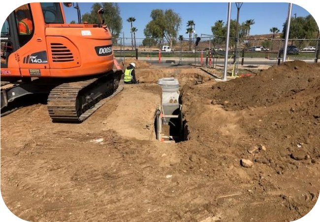
On site manhole installation and backfill
