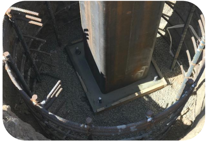
Structural column grouting
