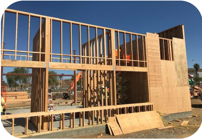
Interior shear paneling installations
