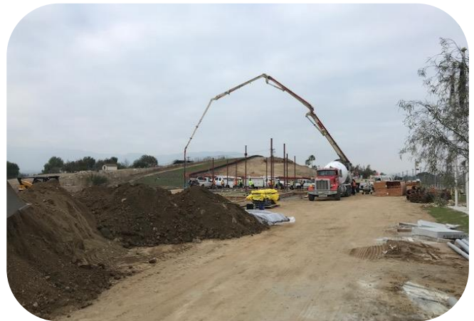
Boom pump concrete placement
