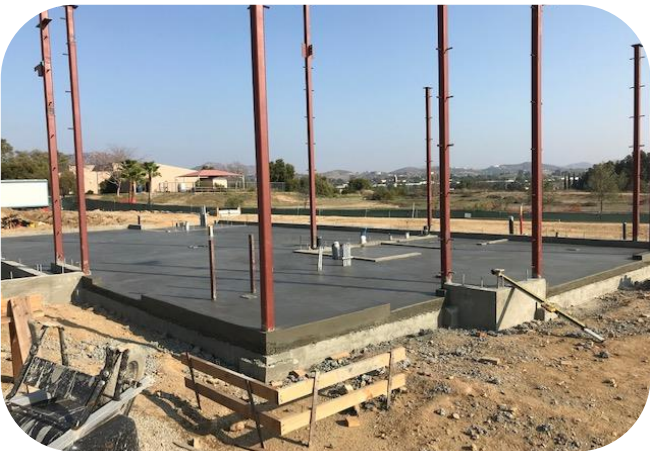
Building Pad Poured
