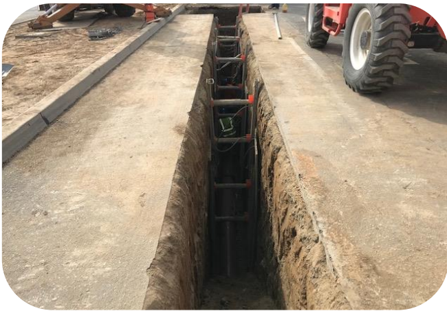
Sewer line to new manhole
