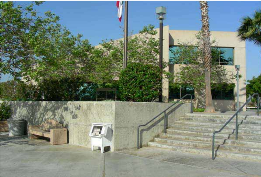
Student Services. This building features odd interior spaces that do not accommodate transformation into multi-purpose classrooms or other flexible space for the delivery of programs and services.
