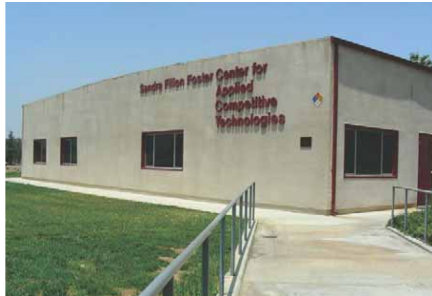
Existing Center for Applied Competitive Technologies (C.A.C.T.). Looking North
