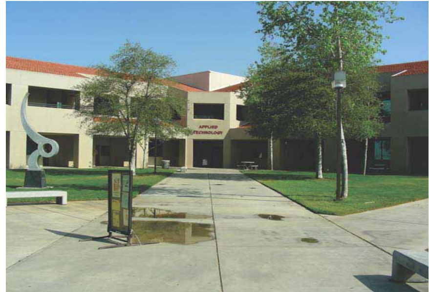
Existing Applied Technology Building. Looking North.
