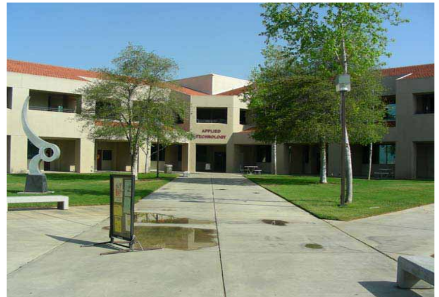
Applied Technology Building. Anchoring the northwest corner of the core campus this building is efficient, understated and in relatively fine physical shape.
