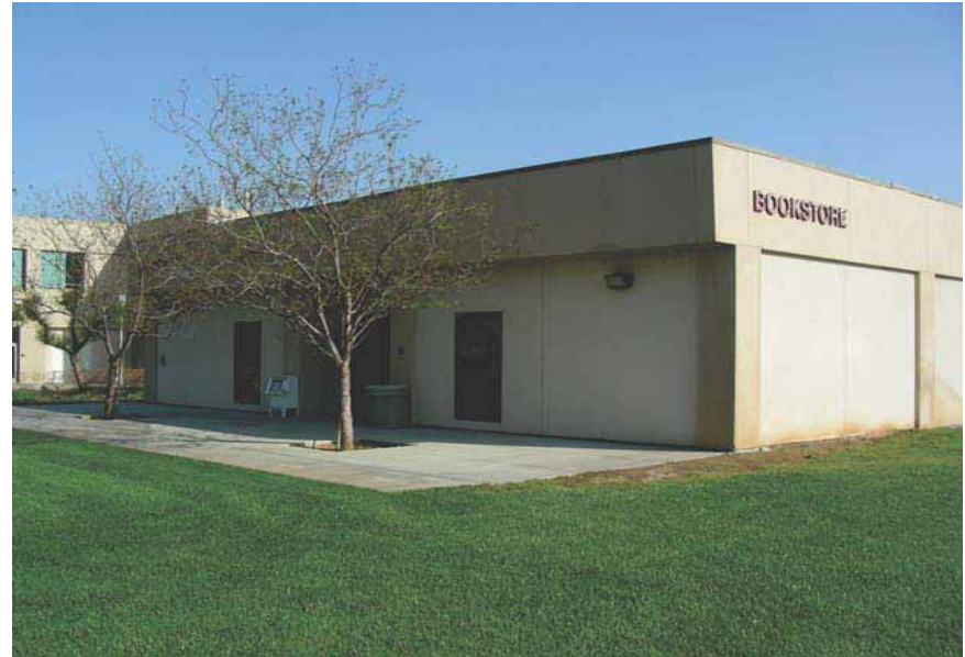
Existing Bookstore. Looking North
