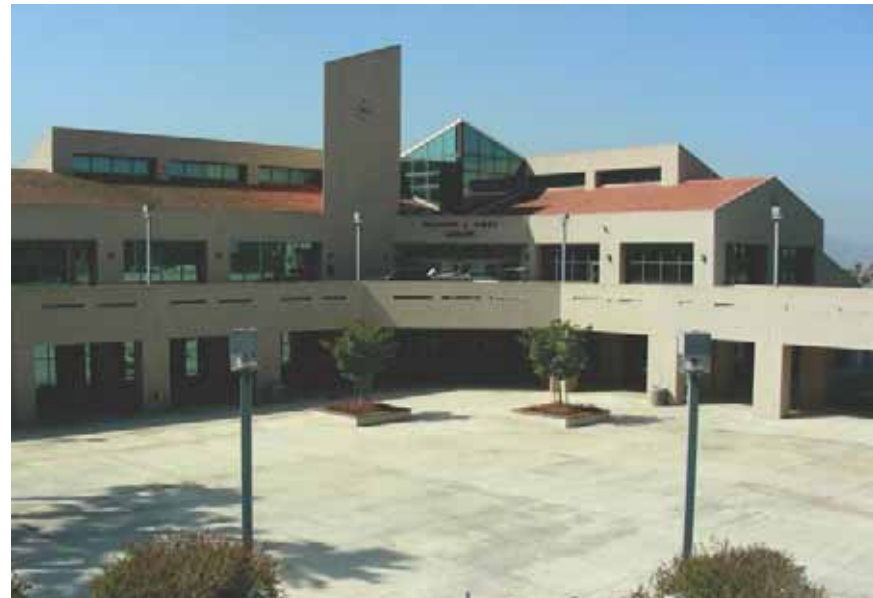
Existing Library Building and Amphitheater. Looking Southwest.
