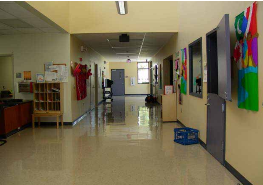
Existing Early Childhood Education Center. Central Corridor
