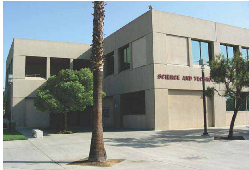
Existing Science and Technology Building. Looking Northwest.
