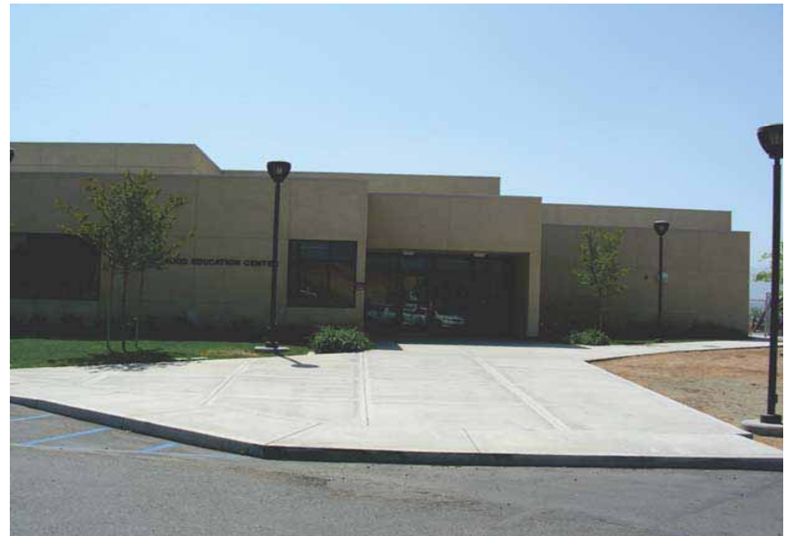
The Early Childhood Education Center. North Elevation and Main Entrance.
