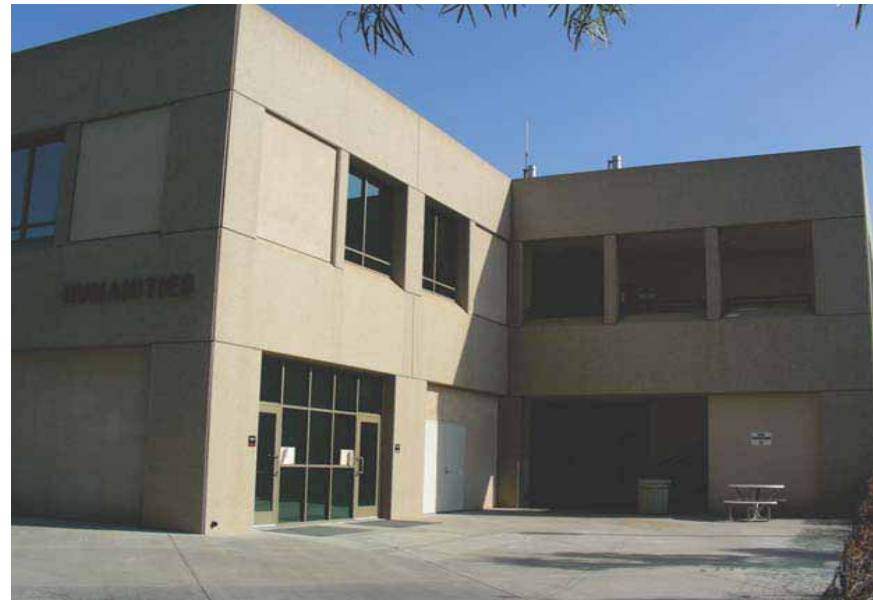
Existing Humanities Building. Looking North.
