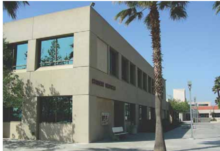
Existing Student Services. Looking Southwest.
