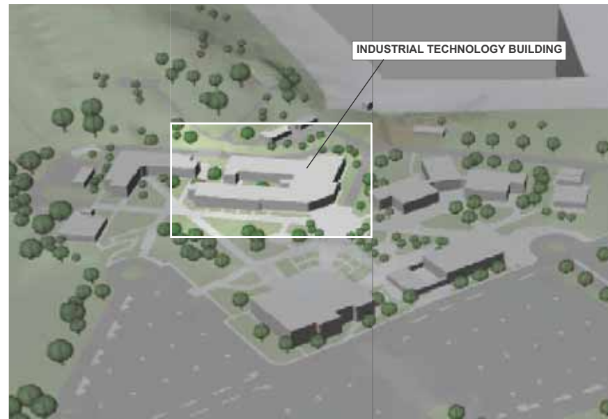
The Industrial Technology Building (Phase III).
